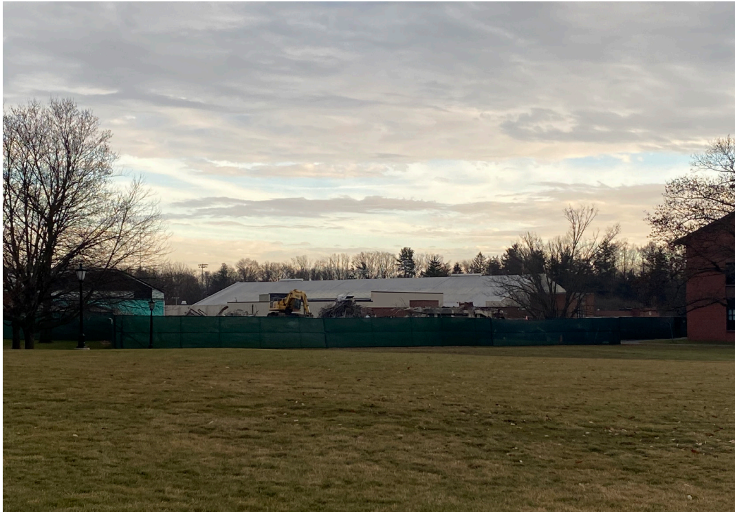
Irwin Dining Hall's demolition process
